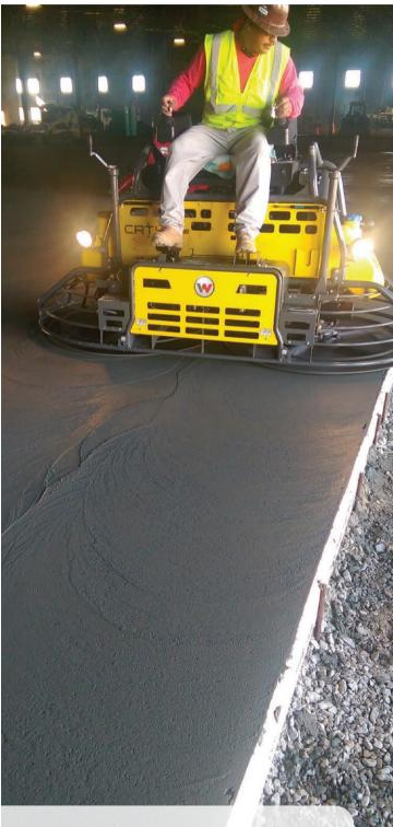
**Intuitive control:** A unique two-joystick electro-hydraulic steering concept on riding trowels allows for precise maneuvers and nearly fatigue-free operation.
