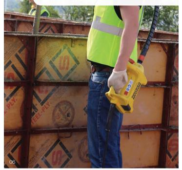
**Making difficult work easier:** The Wacker Neuson external vibration system makes challenging window openings easier to accomplish.
