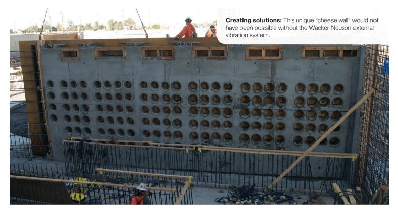
**Get at hard-to-reach places:** External vibration systems mount to wall forms, allowing you to get to places an internal vibrator normally could not.
